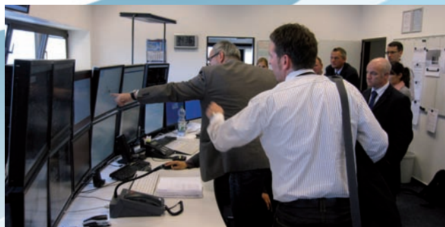
Control room offshore wind farm Alpha Ventus
